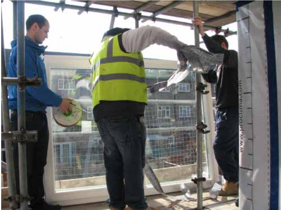
Window installation training at 3 Passfield Drive
