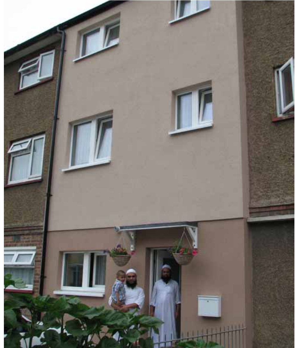
3 Passfield Drive following the Retrofit works
