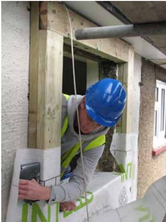
Airtight membranes provide continuity between the window sealing tapes and the parge coat of the external walls
