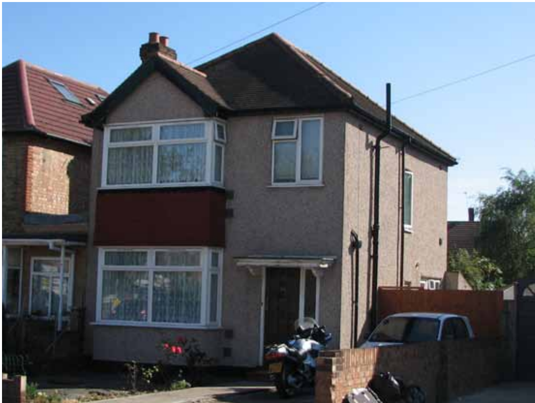
78 Grove Road before the Retrofit works
