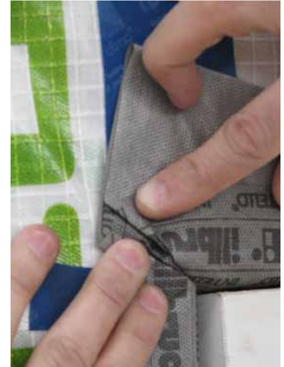
The 'rabbit ears' are folded back so that they can be sealed to the membranes
