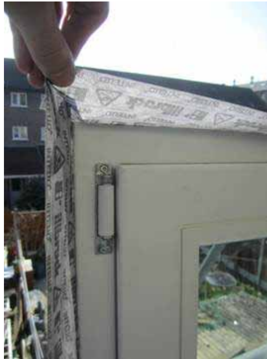
The window sealing tapes are continuous with 'rabbit ears' at the corners to facilitate sealing and allow for differential movement
