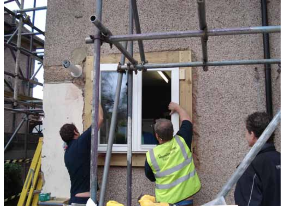
Window installation training at 78 Grove Road
