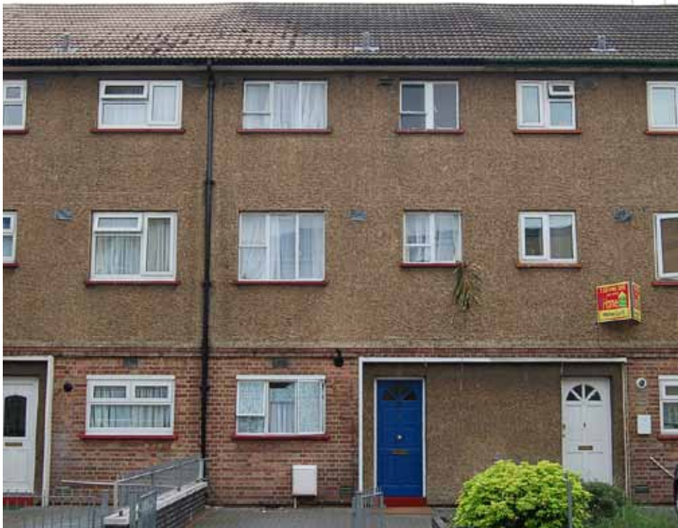
3 Passfield Drive before the Retrofit works
